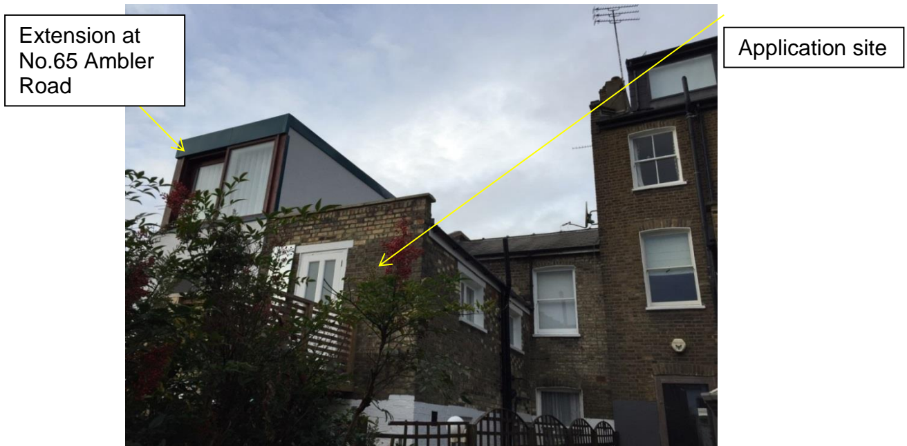
Image 2: View of the rear elevation from No.61 Ambler Road, including the allowed (at appeal) second floor extension at No.65 Ambler Road, the proposed extension at No.63 will be attached to the allowed extension.
